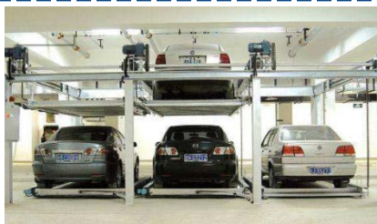
Lift-sliding Mechanical Parking System (PSH)
